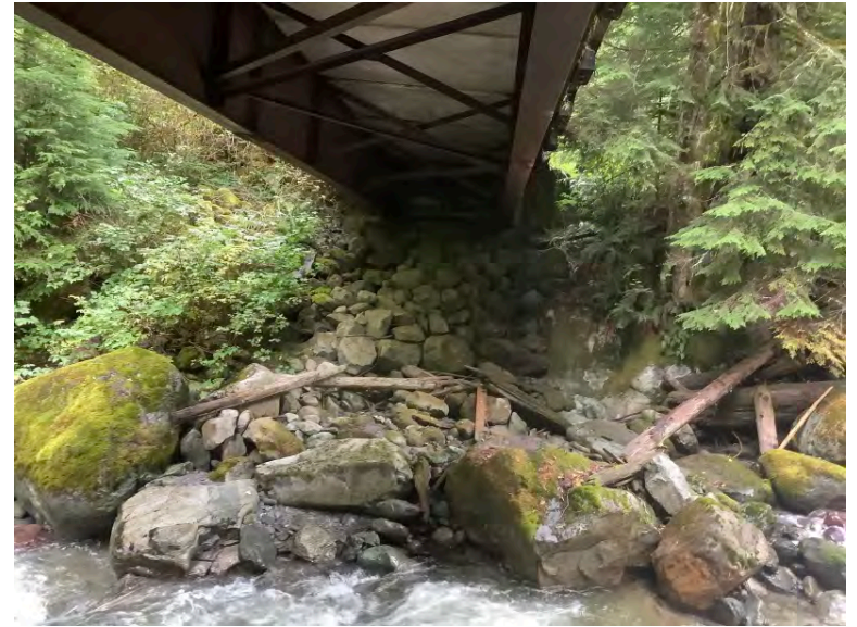
Right Bank Abutment when facing downstream
