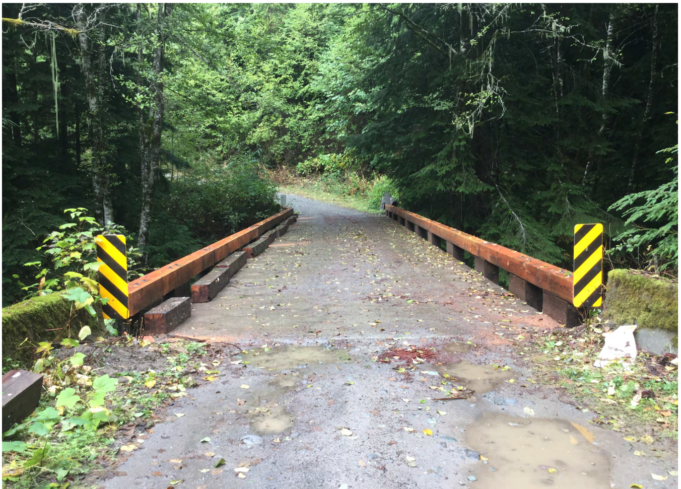
CURBS RECENTLY REPLACED, OCT. 15, 2021
